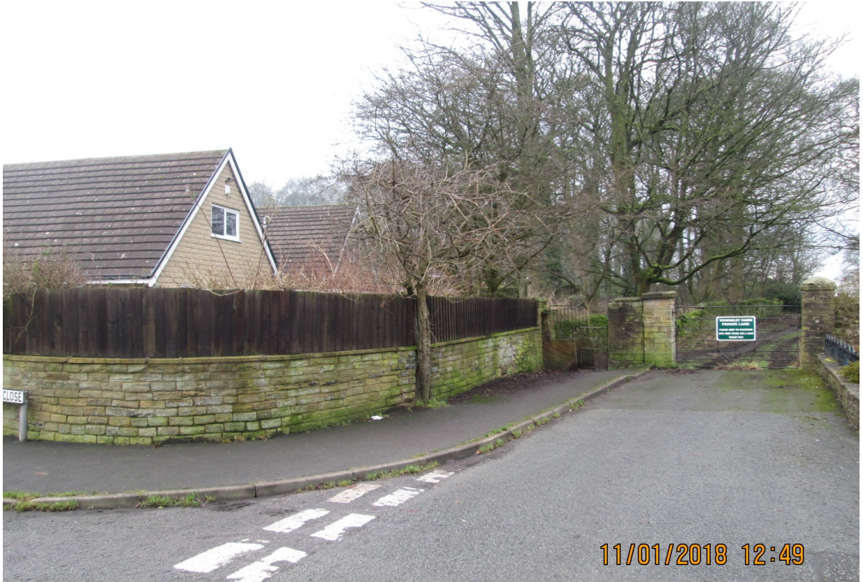
Park Road frontage (rear elevation) and gates to Towneley
